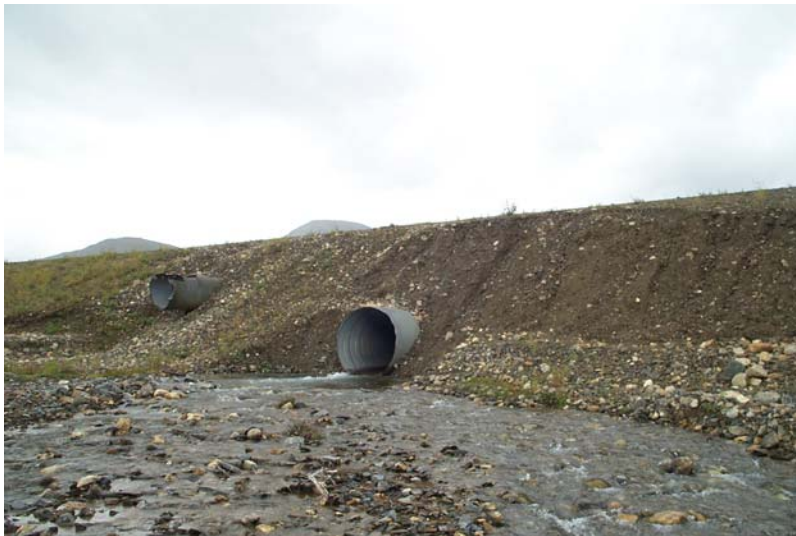
Photo 3. Looking upstream at eroding side slope of Nome-Kougarok Road at Rocky Mountain Creek culvert crossing.
