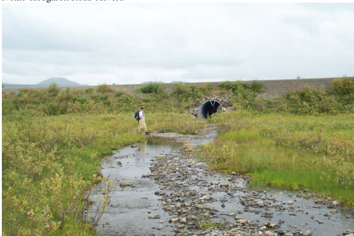
Photo 30. Downstream view of a very disturbed channel in Dexter Creek upstream of culvert in Nome-Kougarok Road.
