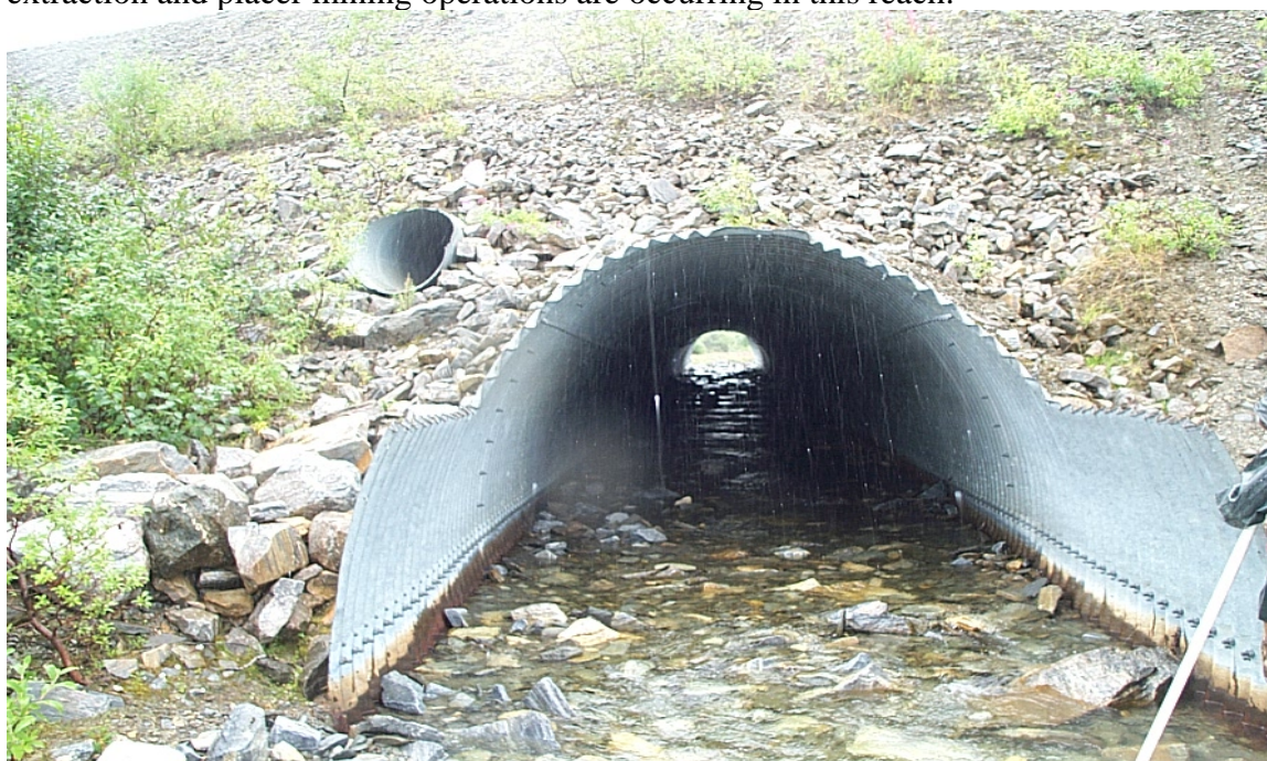
Photo 38. Upstream view of natural substrate in culvert on Sampson Creek. This is a good example of a culvert placement that would provide fish passage.
