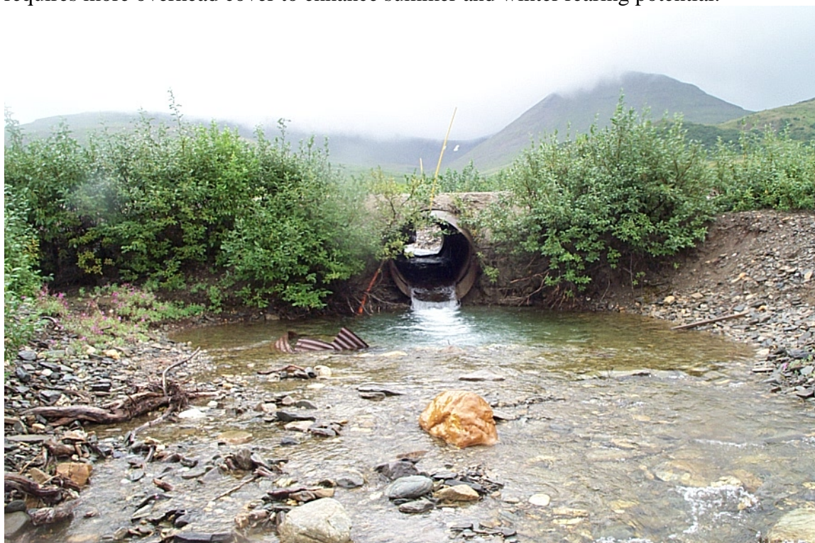
Photo 50. Upstream view of perched culvert (0.30 m drop) at Christian Creek.
